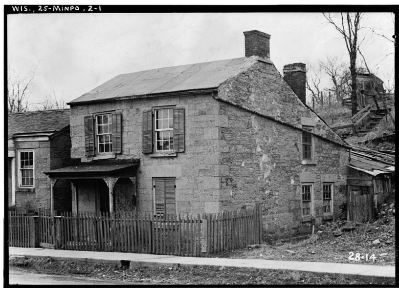
Figure 1: A stone house built by Cornish miners in Mineral Point, photographed for the Historic American Buildings Survey (HABS WI-28-14), Library of Congress. It illustrates the kind of house the Cornish built there; it was not the Penhallows' home.
